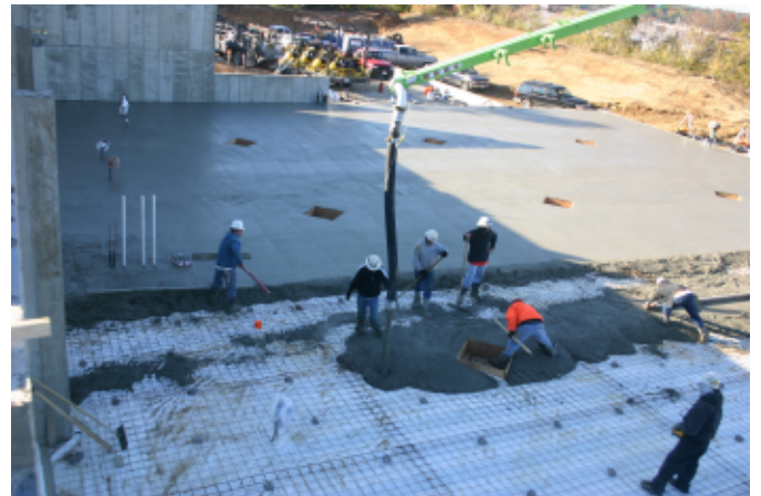
Heating Elements over Insulation and Under 6" Slab
