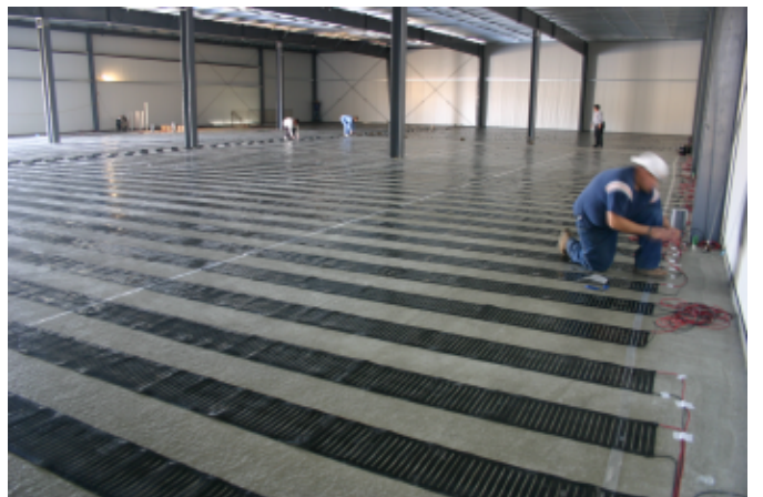
Heating Elements Between Two Layers of Concrete
