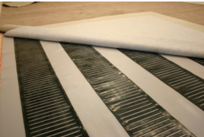
Elements on insulated concrete between two layers of carpet cushion and under carpet
