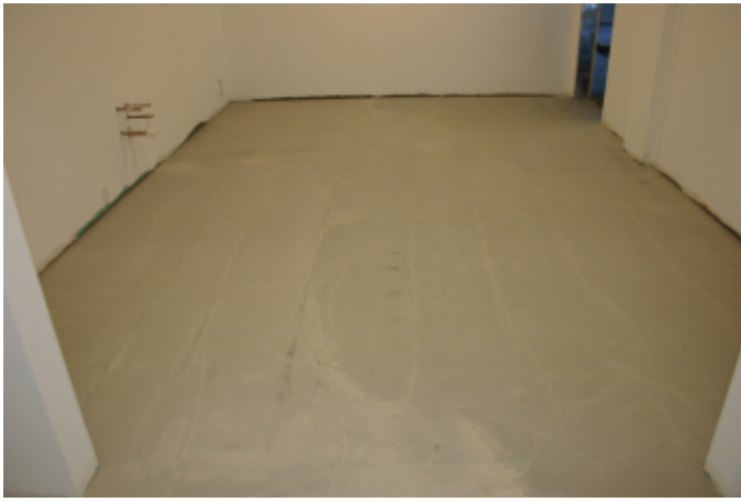
Element Covered by Floor Leveler
