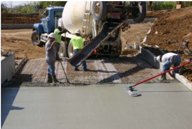
STEP Snowmelt in Vinyl Under Concrete
